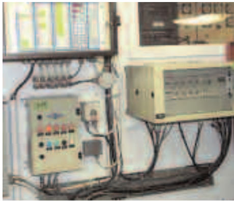
▲ MaK engine controls were easily integrated into the existing alarm and monitoring system. Woodward UG8 MAS governors with 4-20ma speed inputs and rack position sensors allowed an optimised combinator curve with the controllable pitch propellers.
